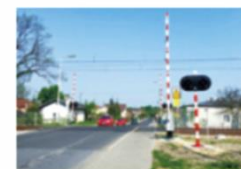
Poland Railway Crossings
